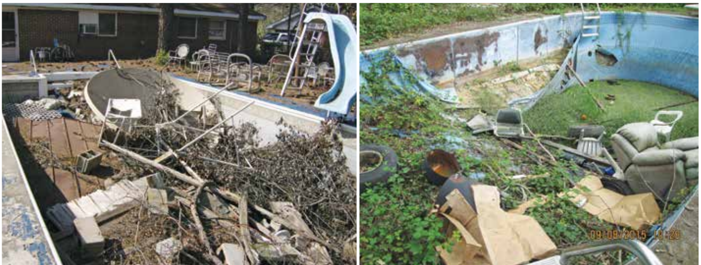
Figure 1: Abandoned pools that require remediation are photographed to document code violations.
